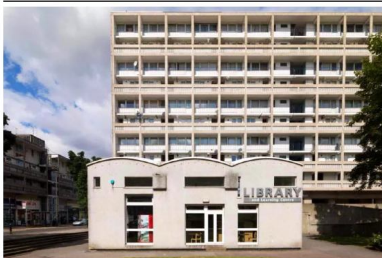
Albrook House and the library, with maisonette blocks over shops to the left. Every building in this photo is proposed for demolition. Photo: James O. Davis/Historic England
